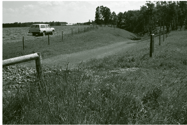
Figure 8.3.3 Constructing Grassed Waterways.
